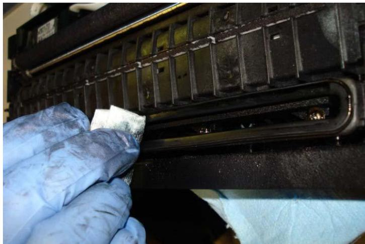
*Picture of wiping the Cap Seal with damp lint-free cloth*
